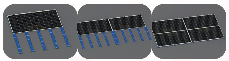
Gluing at the ribs of the CS support, installing and flattening the assembly, placing the junction box side at the service walkway, and rolling the surface of the module with a plastic roller to ensure a good bond between the module and the CS supports.
